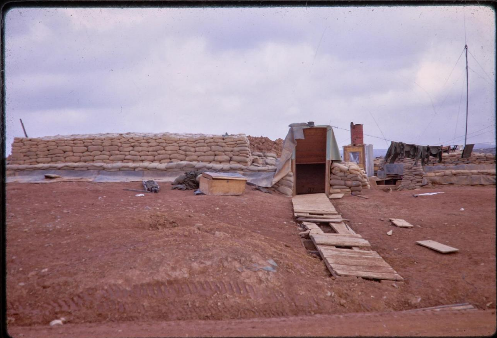
Medical staff housing reinforced by layers of sand bags
