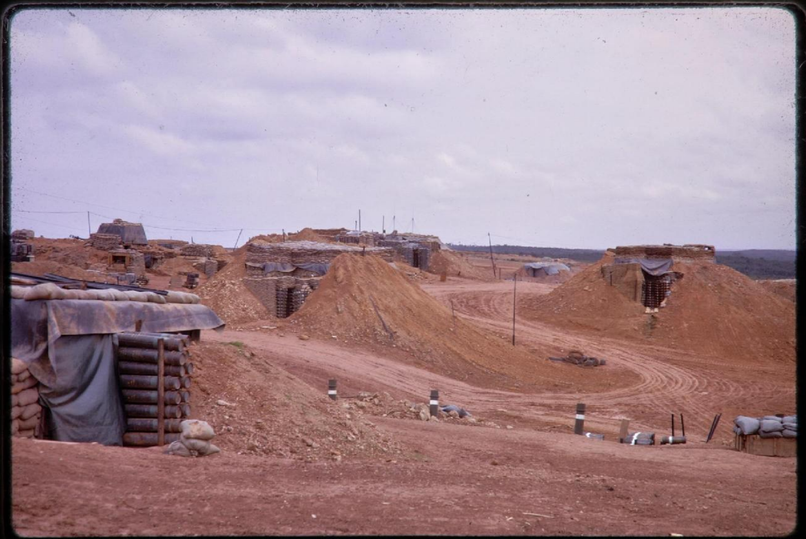
Bunkers constructed of very heavy timber framing supporting layers of sandbags to prevent artillery shells from penetrating
