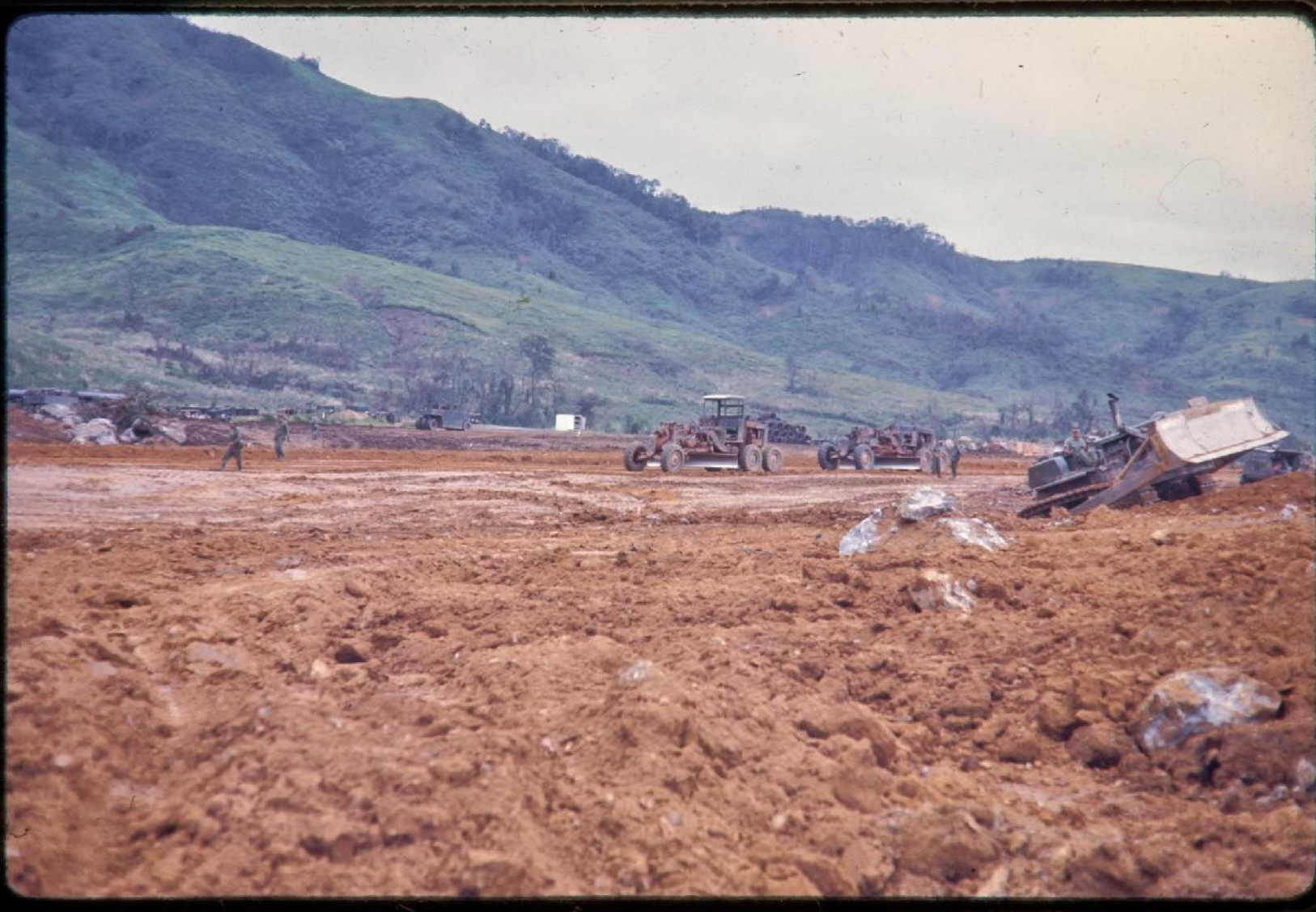
Seebies begin construction of airfield to receive supplies to rebuild the road to Khe Sanh
